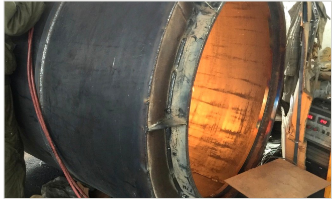
02 Shop floor · large-diameter circumferential welding
